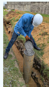
CATHODIC PROTECTION WORKS
