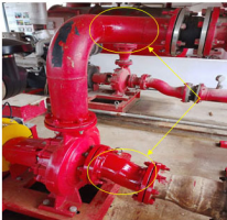
Modifications to the intake/discharge lines of the new DCI motor-pump unit.
