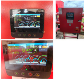
Installation, connection, power-up, configuration and commissioning of the new DCI motor-pump unit.
