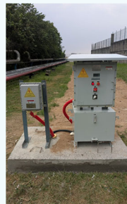
CATHODIC PROTECTION WORKS
